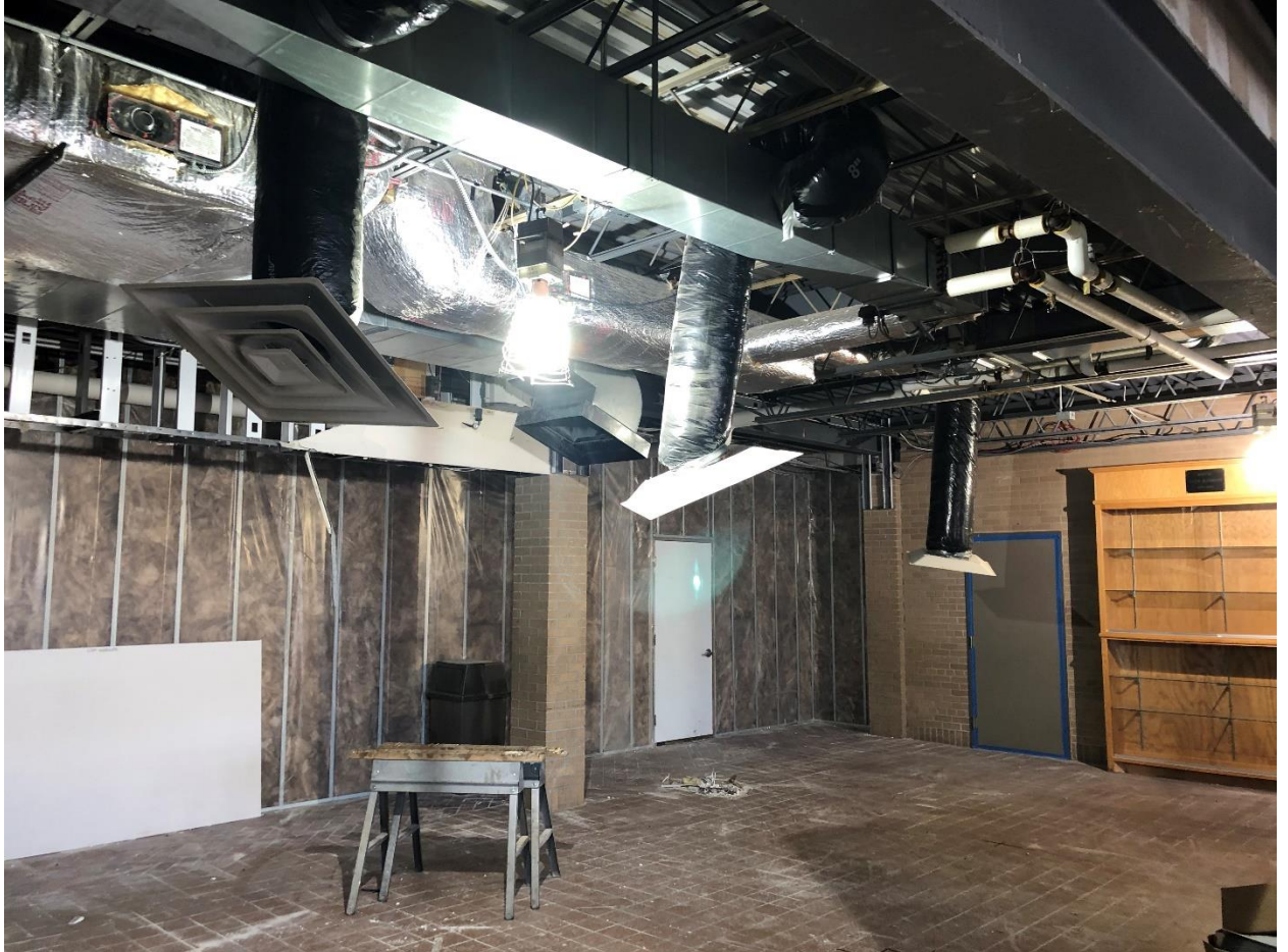
High School/Middle School Commons: Mechanical and Electrical demolition
