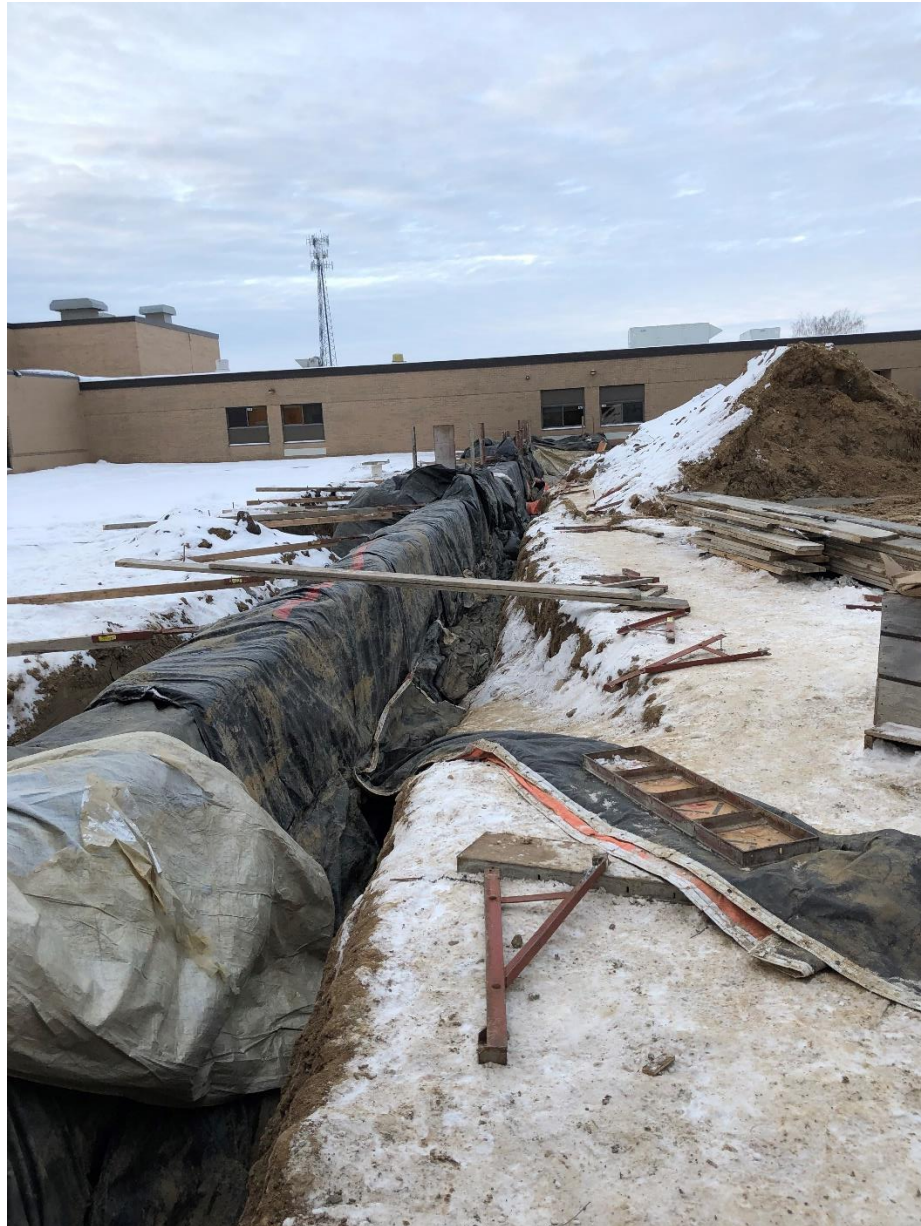
Elementary School Addition: Blankets over concrete foundations
