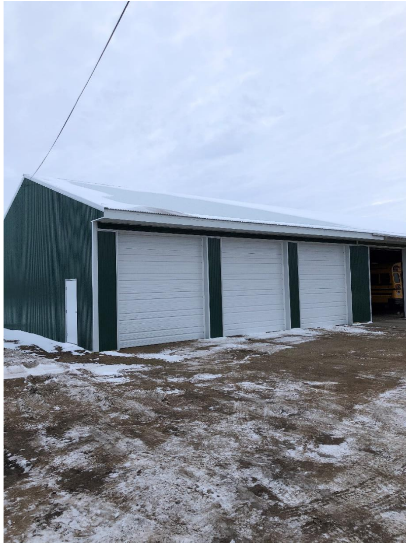
Transportation Building: Garage doors installed
