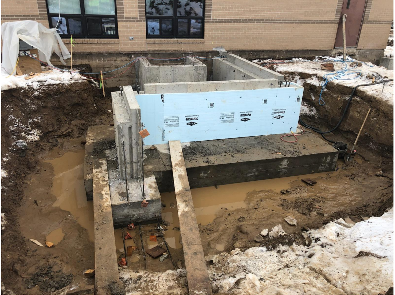
Elementary Classroom Addition: Footings/Foundation poured
