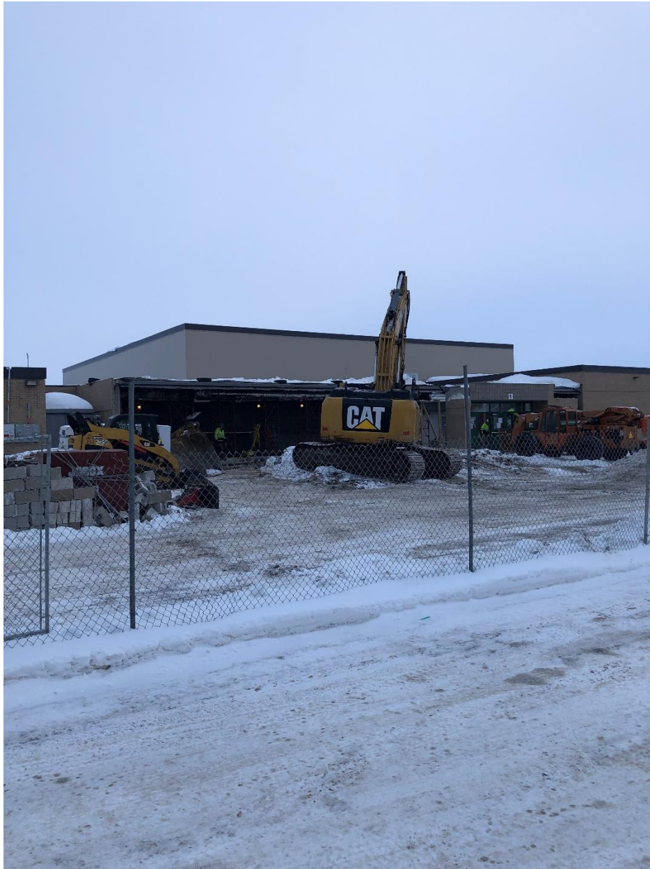
High School/Middle School Additions and Renovations: Demolition and Shoring exterior wall
