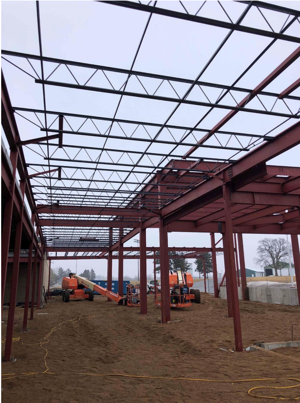
High School/Middle School Commons Addition: Joist installation, Decking to follow
