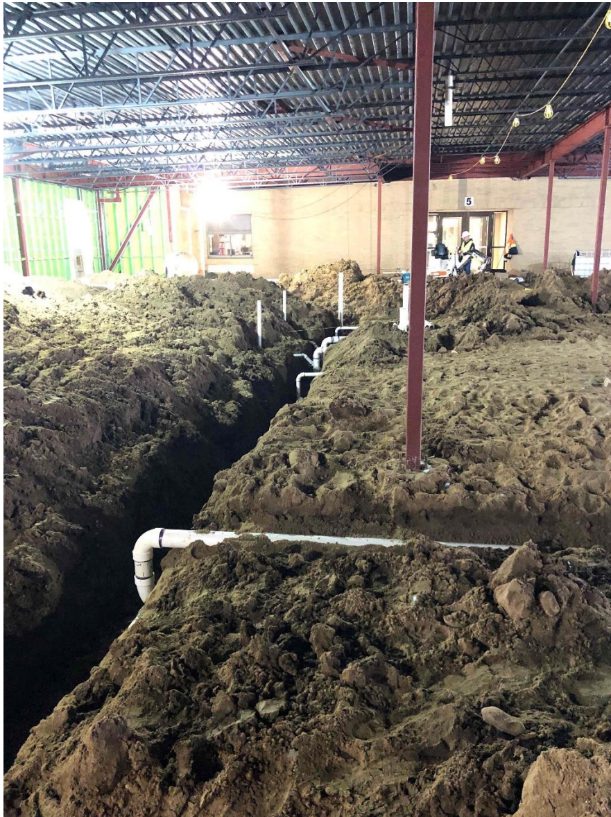
Elementary Classroom Addition Underground plumbing, backfill and concrete slab to follow
