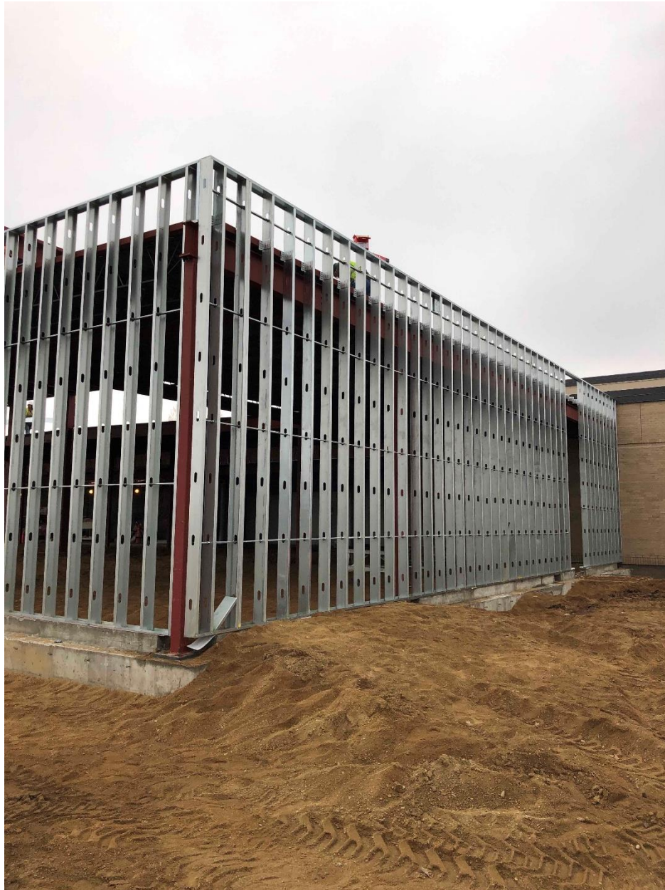
High School/Middle School Commons Addition: Exterior steel studs installed
