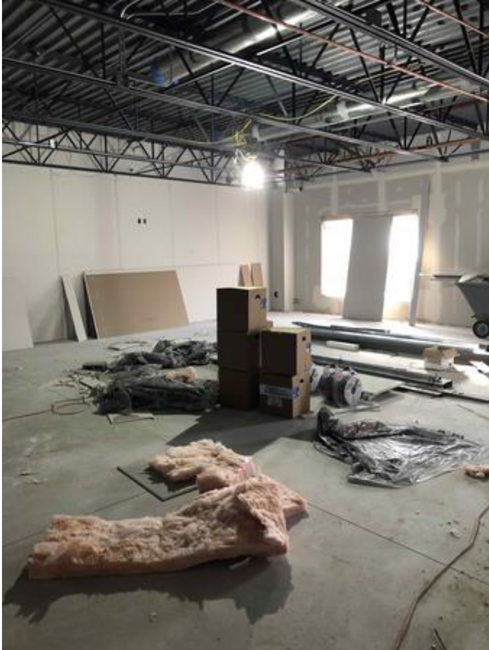
Elementary Classroom Addition Sheetrock continuing in elementary classrooms
