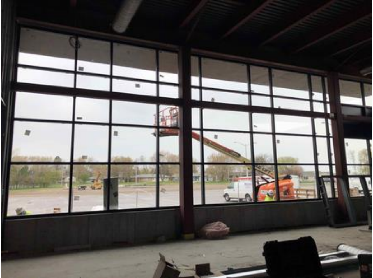
High School/Middle School Commons Addition: Windows installed at front entry
