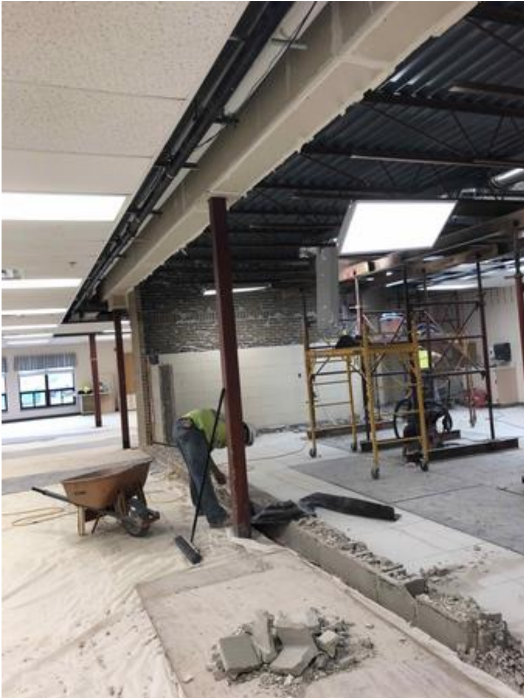
Cafeteria Remodel: Shoring up, demo ongoing in cafeteria
