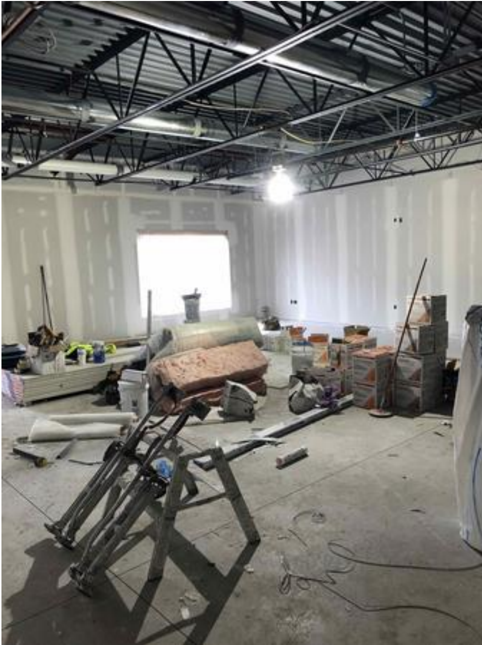
Elementary Classroom Addition: Drywall and taping complete in classrooms
