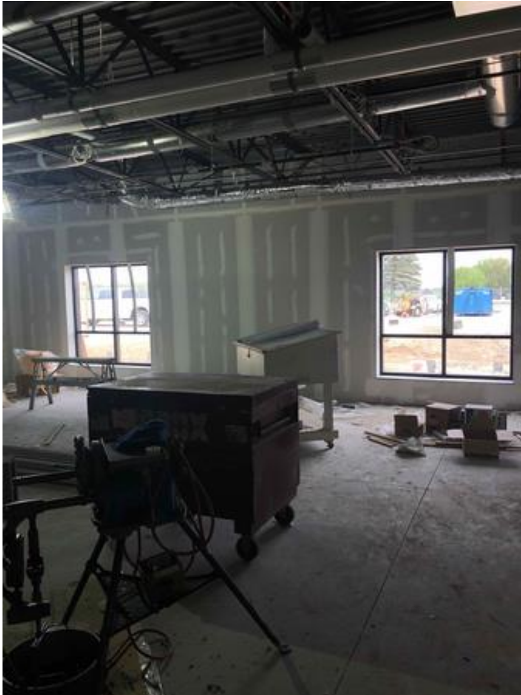
Elementary Classroom Addition: Windows installed, painting and acoustical ceilings to follow
