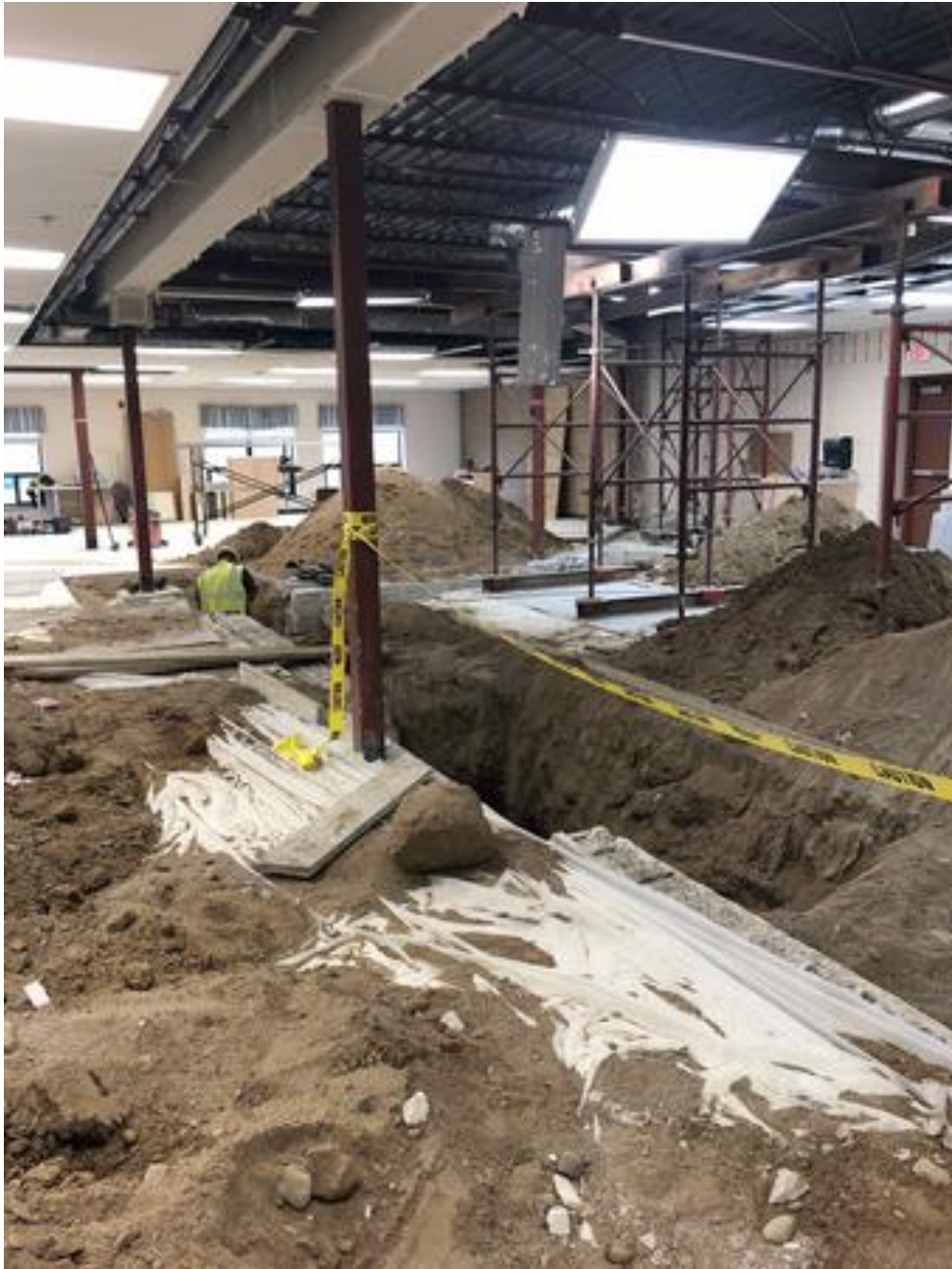
Cafeteria Remodel: Demo complete, concrete foundation to follow
