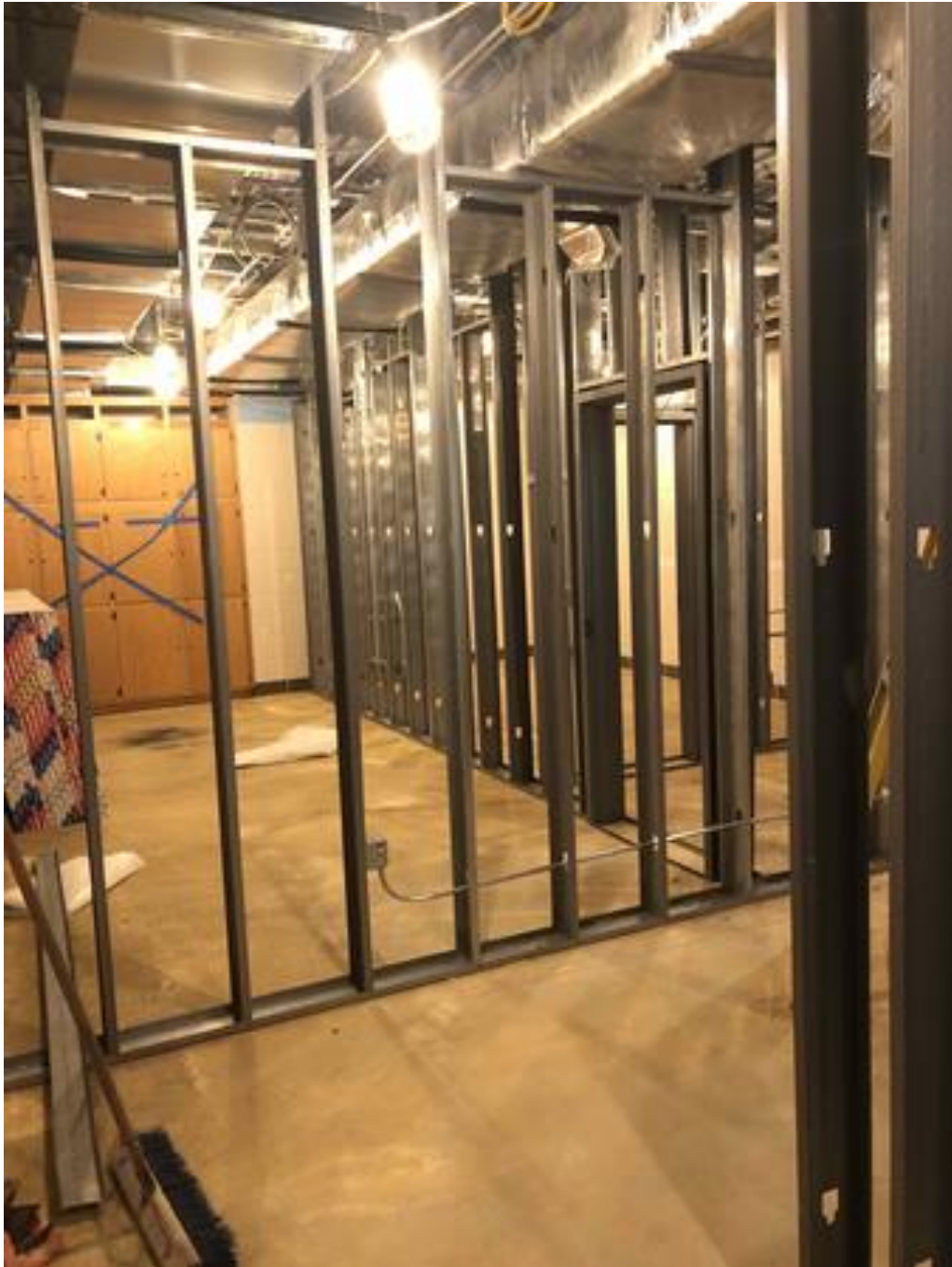
Team rooms/offices: Framing complete in team rooms, drywall to follow
