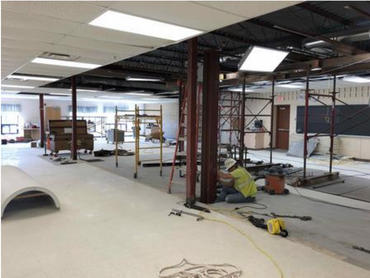
Cafeteria Remodel: Demo complete, installaing structural columns. Soffit framing to follow
