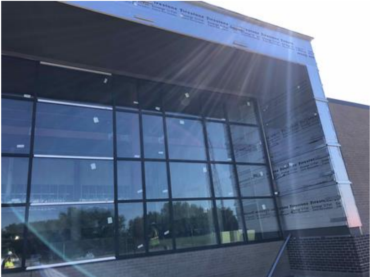
High School/Middle School Commons Addition: Metal panel insulation ongoing
