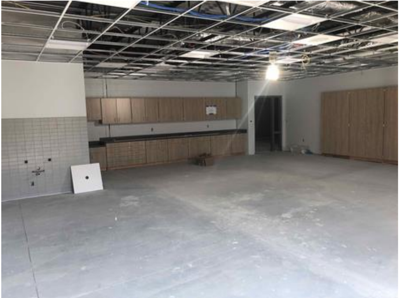
Elementary Classroom Addition: Casework and tile complete
