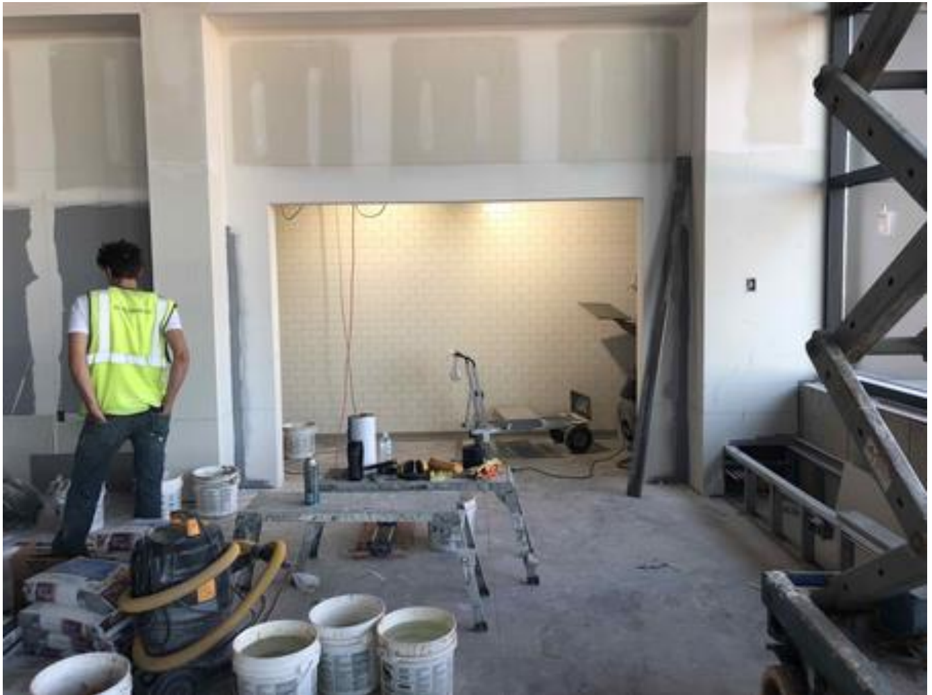
HS/MS Renovations and Additions: Tile walls and floors ongoing
