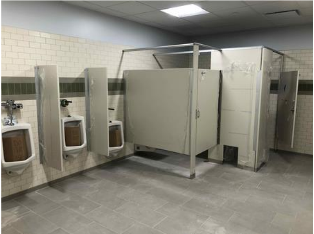
High School/Middle School Commons Addition: Restroom fixtures complete
