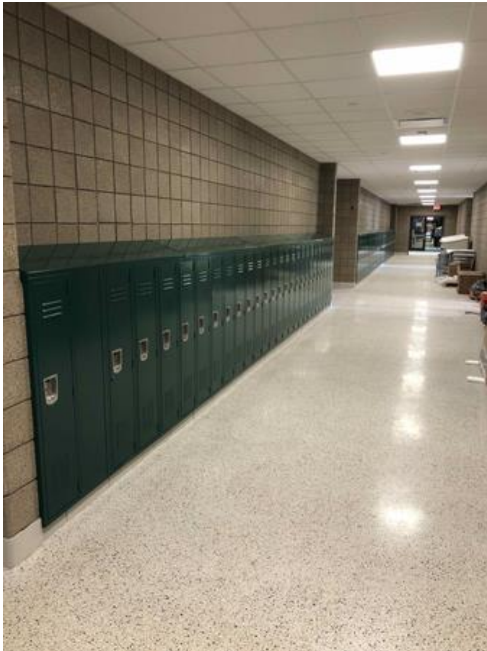
Elementary Classroom addition Lockers complete
