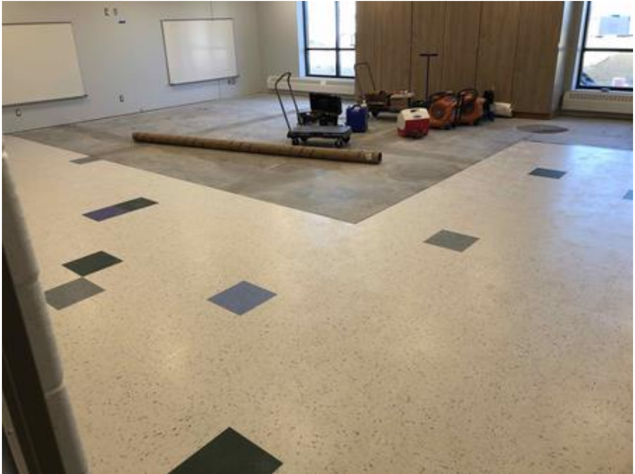
Elementary Addition: Elementary flooring ongoing
