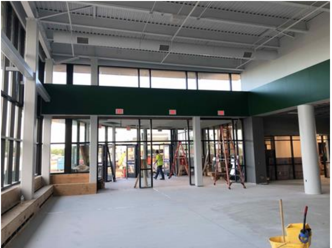
HS/MS Renovations and Additions: Painting, glass, exit signage, HVAC etc. complete
