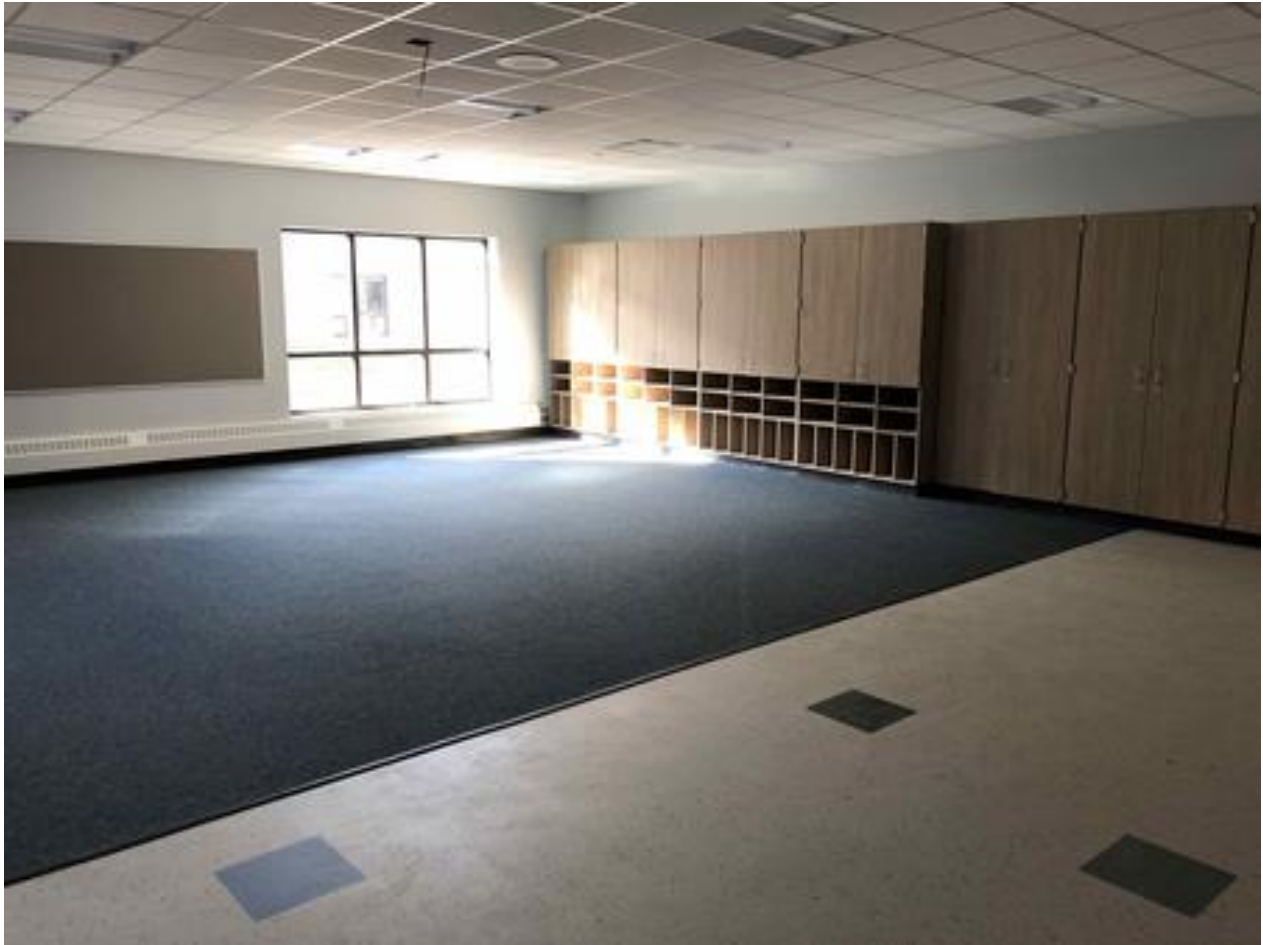
Elementary Classroom addition Flooring Complete
