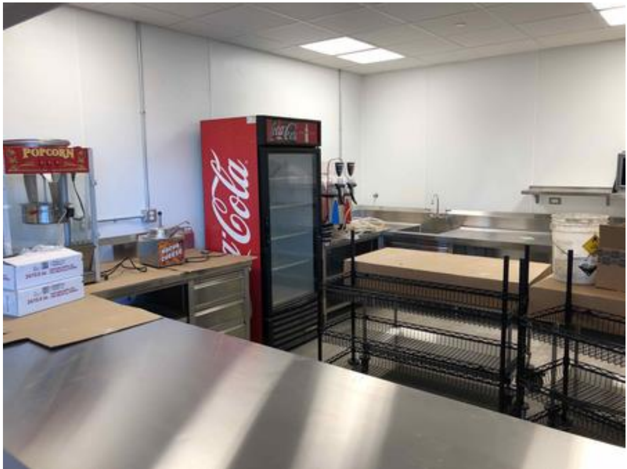
HS/MS Renovations and Additions: Concession stand equipment installed
